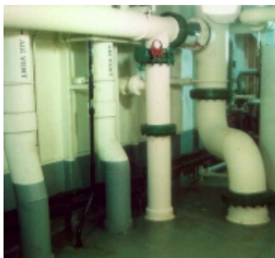
BELZONA® 5131 REDUCED CONDENSATION ON THESE COLD WATER PIPES
