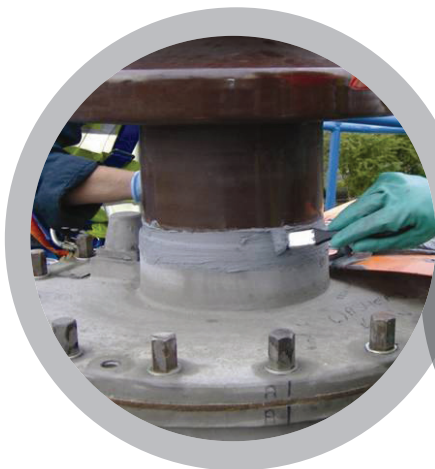
Joint Sealing
