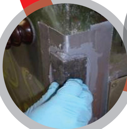
Cold Plate Bonding
