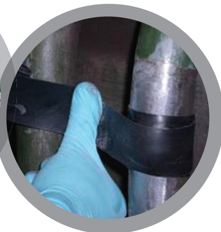
Oil Leak Repair
