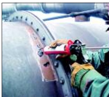
INFILL CORROSION PITS
